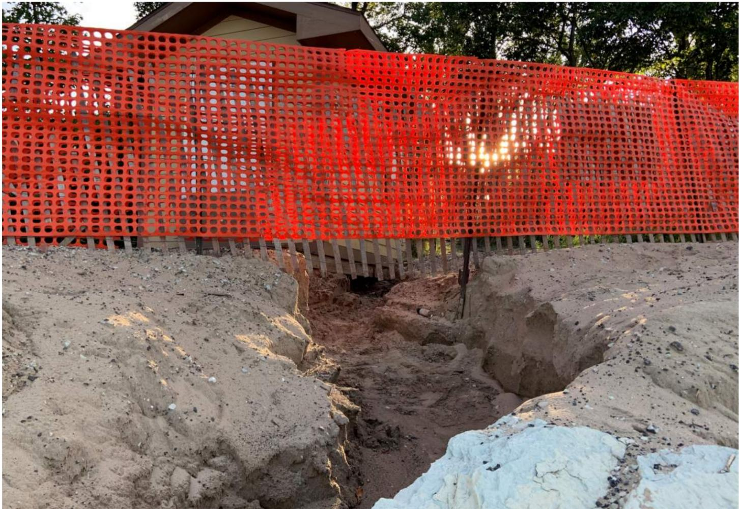
Stormwater running down the slope led to erosion under the building. The building has been removed. (2019)
