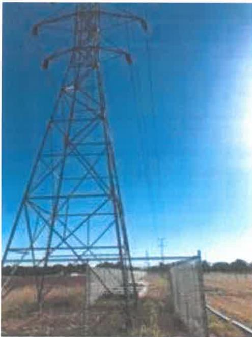
*So one of the first things we should notice prior to starting each job is hazards such as this one that require addition communication with a jobsite superintendent or in this case the power company to either insulate or shut off the power to these lines.*
